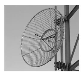
mWAVE supports all current and legacy Mark parabolic grids with feeds, wind brace kits and other miscellaneous parts and tuning services.
